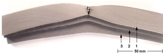
Fig. 8: Cross Sections Through the Crack in the Metallic Shell of the Transfer Line
